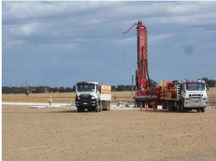
Figure 27: Production bore drilling underway. Note young saltbush Plantation in background.
