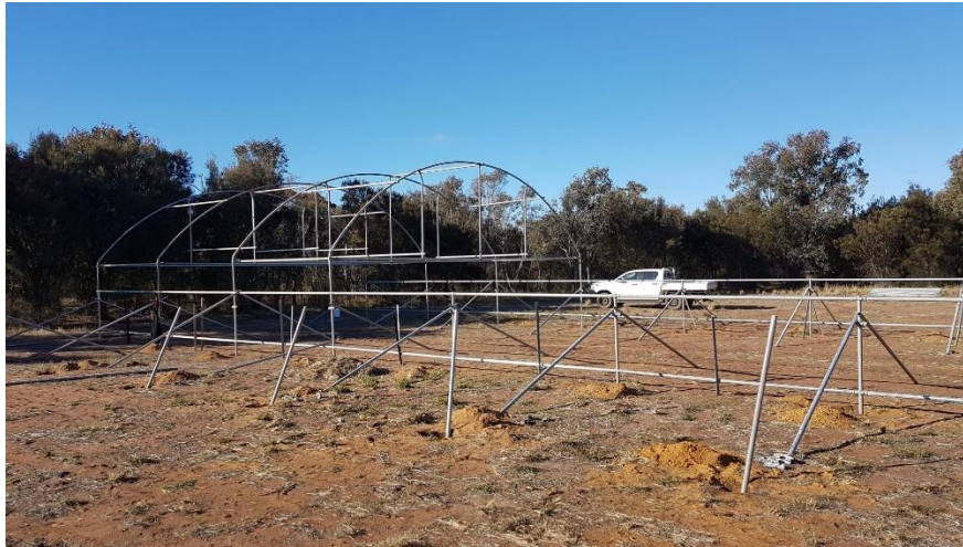
Figure 21: Shadehouse 1 under construction.
